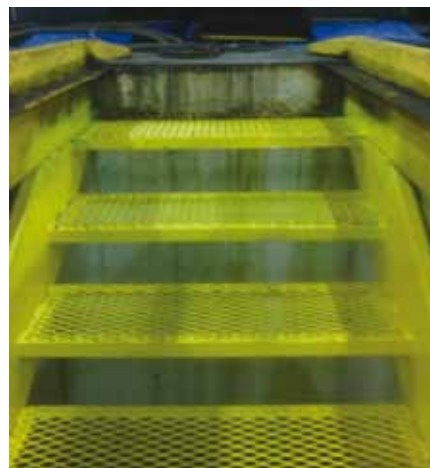
Newly built stairs installed
